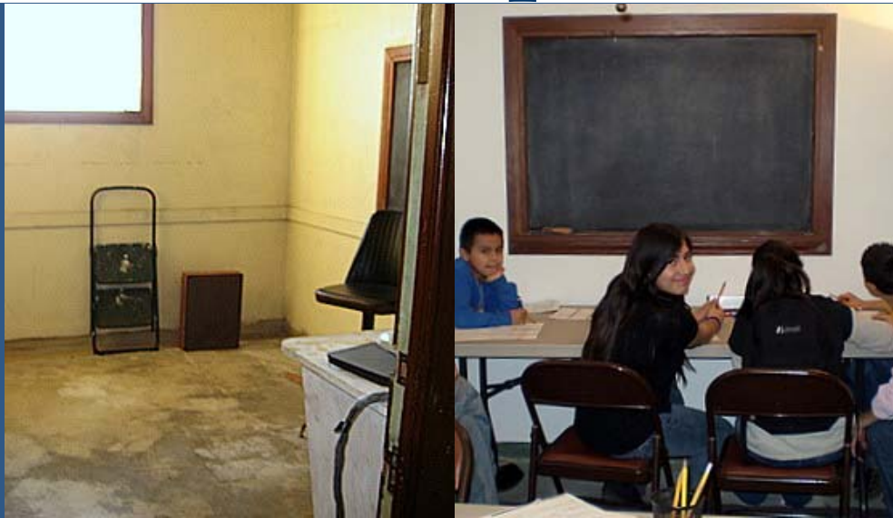
A renovated classroom- before and after.
